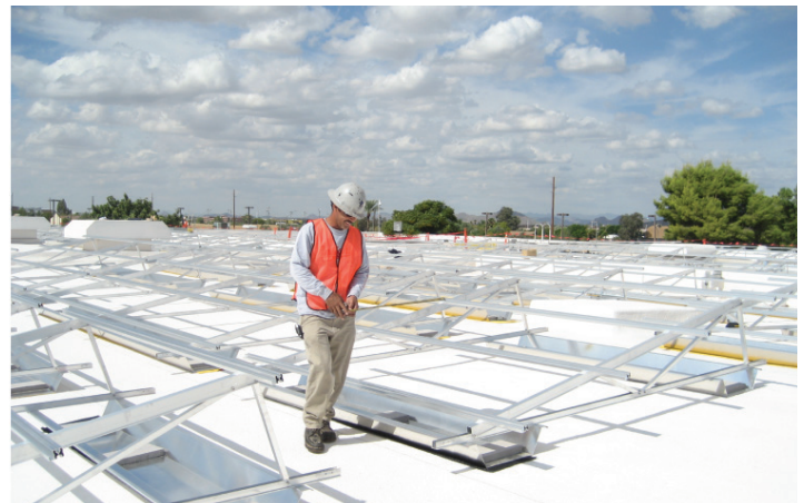
Non-penetrating Windsafe installation
