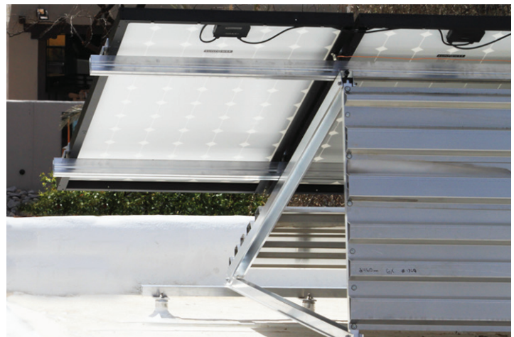
Penetrating Windsafe installation
