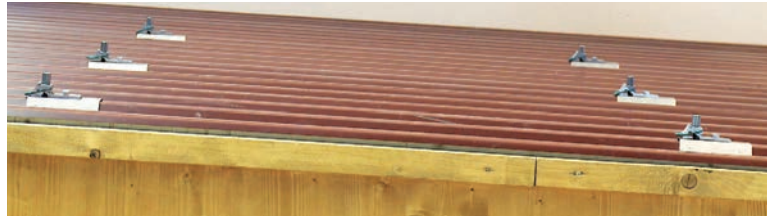
roof attachment example shown is for Fix2000
