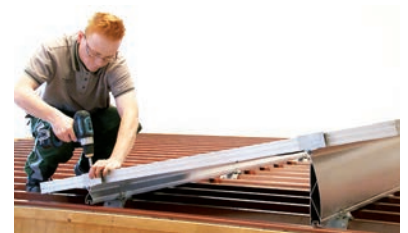
❸ Install modules
